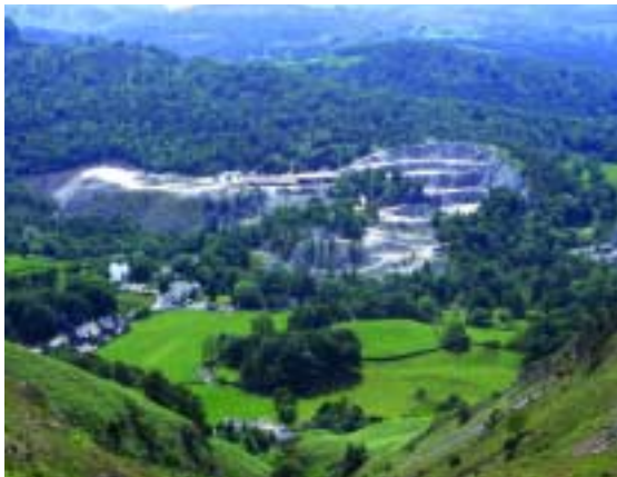
Elterwater Quarry, Lake District. An acceptable modern scheme was agreed at this sensitively located slate quarry.
